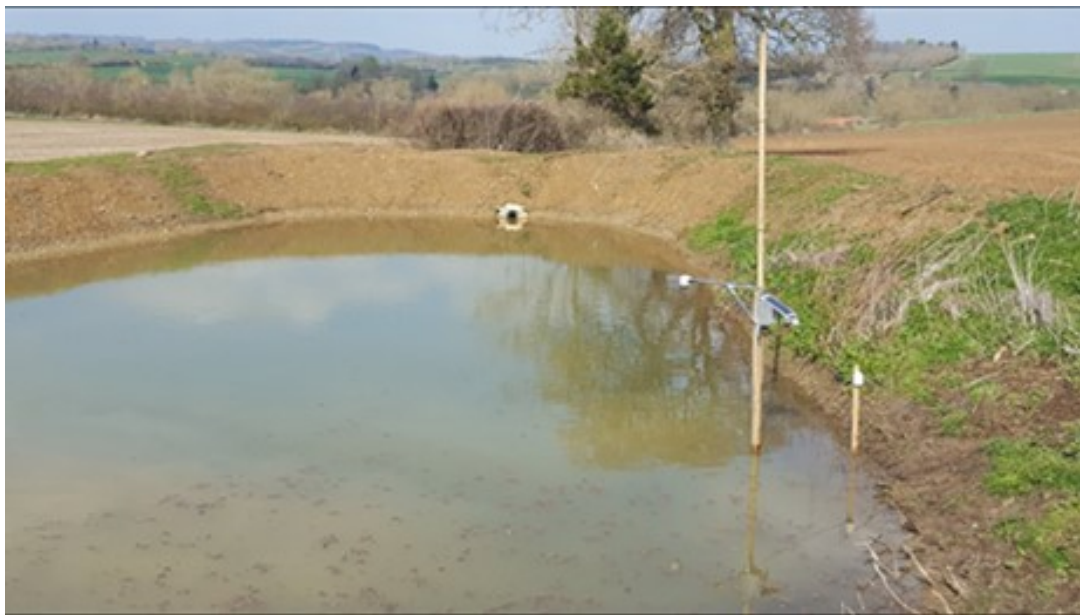
Figure 23 Farm retention pond with drain in Stour river catchment with water level and soil moisture sensor.
